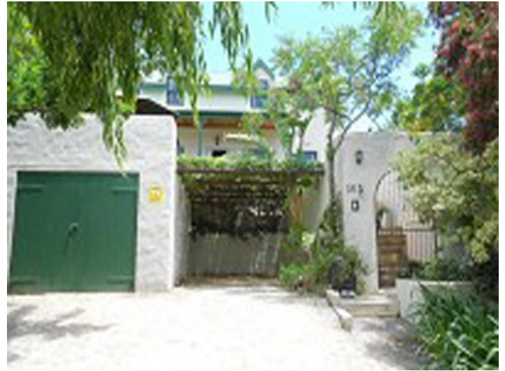
Entrance and garage of the property
