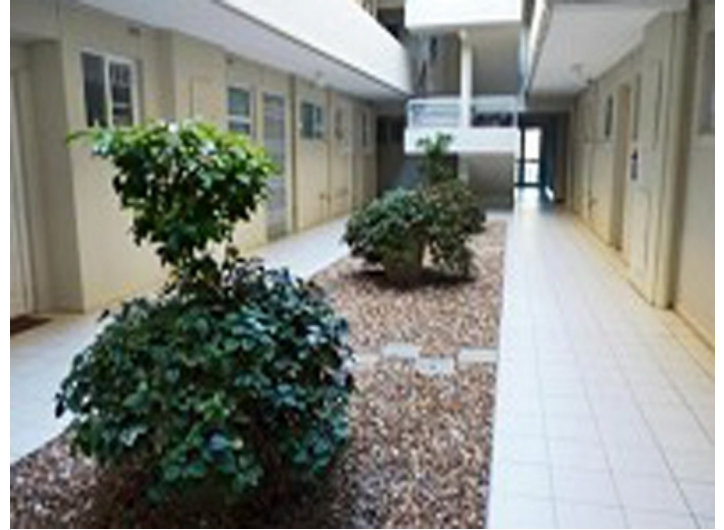
The rest area inside the block
